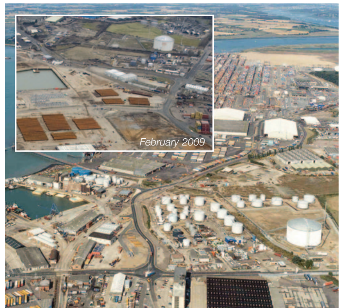
The tank farm in its heyday
